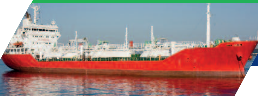
Seawater cooling pipelines on board deepfreeze stern trawler Carolien
