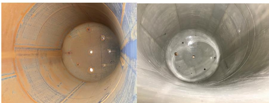
**FIGURE 3** Before (left) and after (right) lining a steel tank with PVDF copolymer sheets. Images courtesy of Electro Chemical Engineering & Manufacturing.
