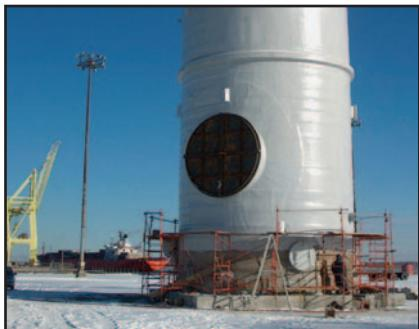
Steel blinds were made to allow pressure testing of the scrubbers at the port.
