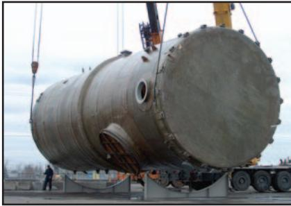
After assembly at the port, the scrubber is moved for pressure testing.
